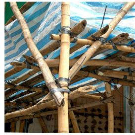
On the major high-rise buildings the bamboo poles near the bottom have to be large to support the weight. Here is an example of how the bottom poles look in one of those applications.
