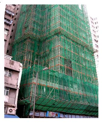
The bamboo poles are bound together with a high strength polymer twine. This seems like a positive move from the hemp or other natural fiber they probably used for this purpose in 1959 and before.
